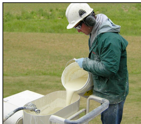
Supplied as a white, food-grade powder, ORC® is usually mixed with water on-site and placed into the subsurface by direct injection.
