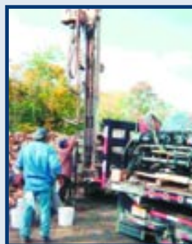
Bedrock Injection with Inflatable Packer System
