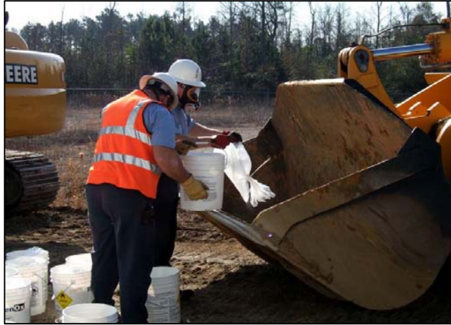
Figure 2: Application of RegenOx with a Front End Loader.
