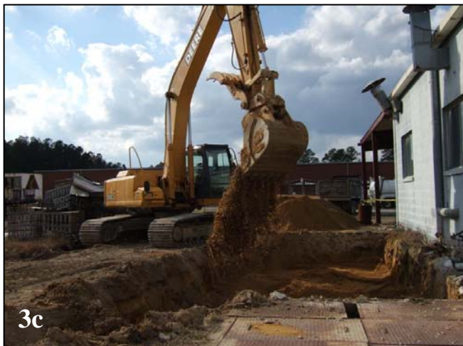
Figure 3: Photo Documentation of a RegenOx Excavation Application.
