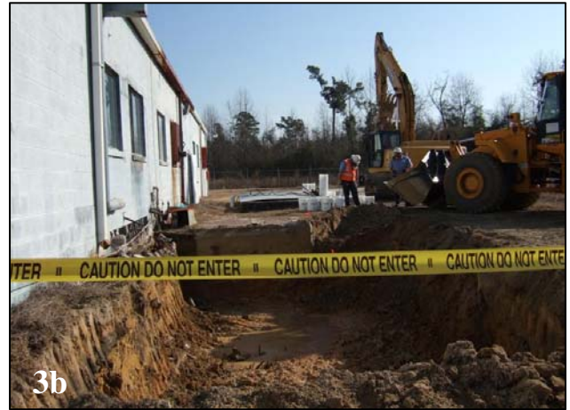
Figure 2: Application of RegenOx with a Front End Loader.
