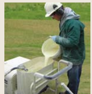
FIGURE 1: FILLING A PUMP WITH ORC ADVANCED SLURRY
