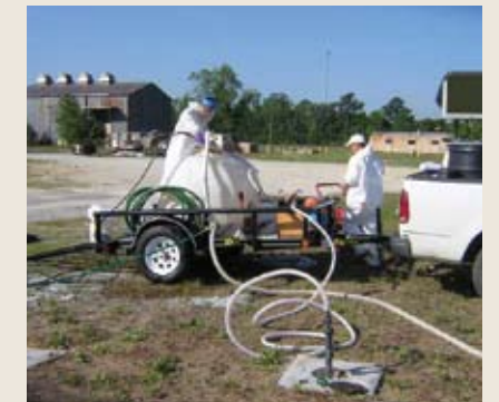
3-D Microemulsion is typically applied through permanent wells or by using direct-push injection.
