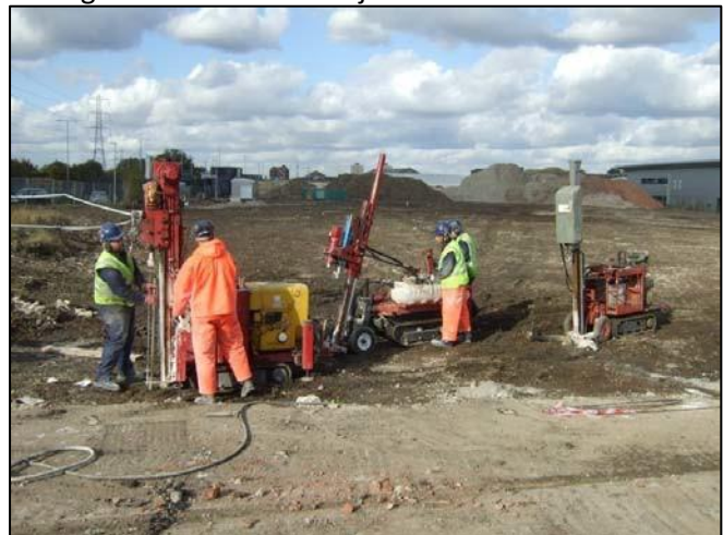
Figure 1. Direct-Push Injection of ORC Advanced®
