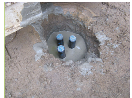
Fig.4: Nested injection wells as built
