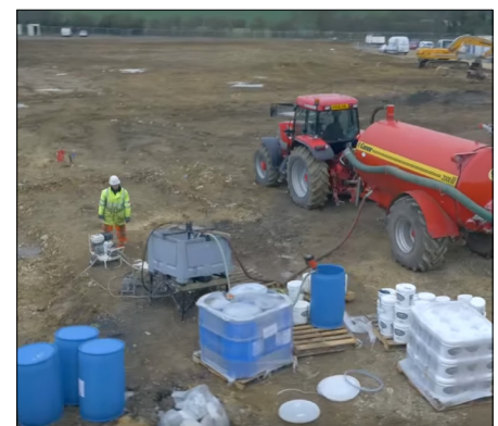
Fig. 1 and 2 - REGENESIS carrying out the injection of MRC and 3DMe on site
