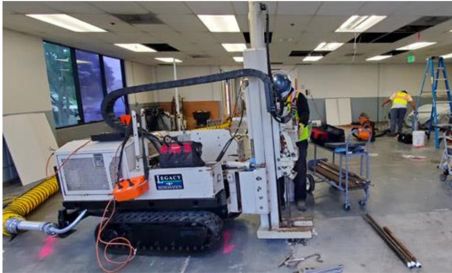
Figure 5. Injections in the building office area at AOC-1.
