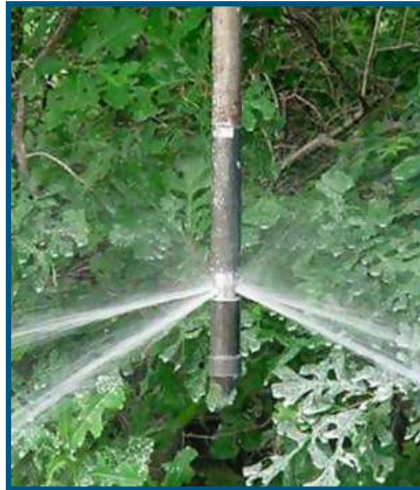
FIGURE 6 Image of Geoprobe ® pressure activated injection probe
