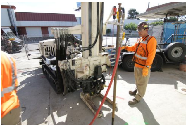
REGENESIS Remediation Services mix and monitor remedial amendments in a services trailer onsite (top). Then the remedial amendments are placed in situ using a GeoProbe (bottom).
