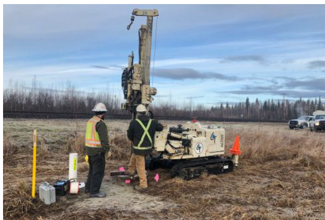
A field application on a U.S. airport uses a colloidal activated carbon (CAC) barrier to address PFAS groundwater impacts caused by an aqueous film forming foam (AFFF) concentrate, a firefighting foam being phased out of use due to its high levels of PFAS.
