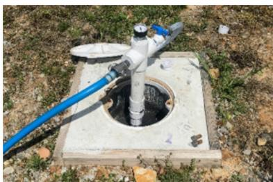
*A recommended well head injection fitting system that has an inlet, pressure gauge, and outlet.*
