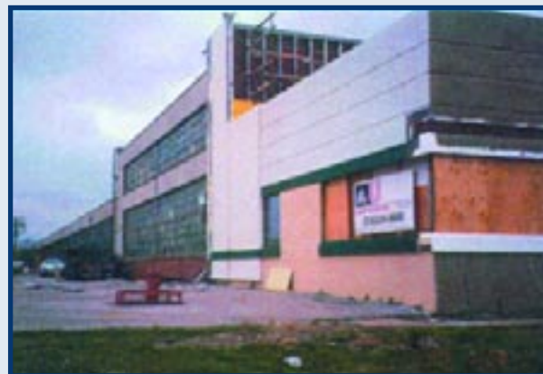
Site after cleanup and development
