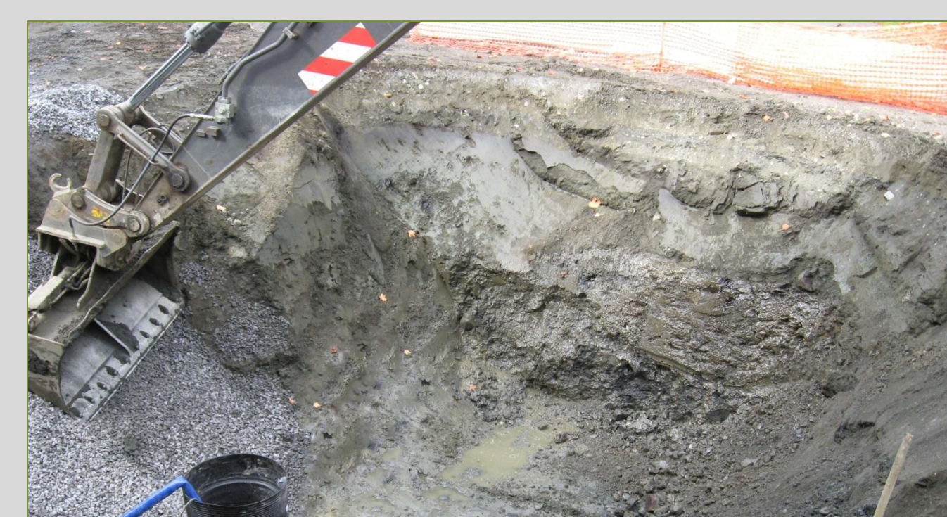
Application of RegenOx to Sidewalls and Base of Excavation
