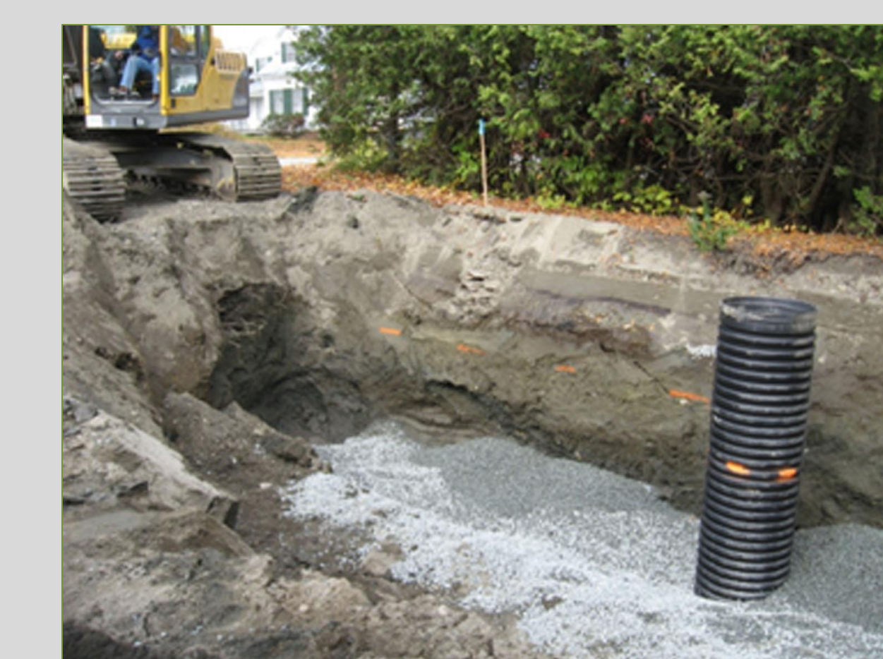
Interceptor Trench Installation
