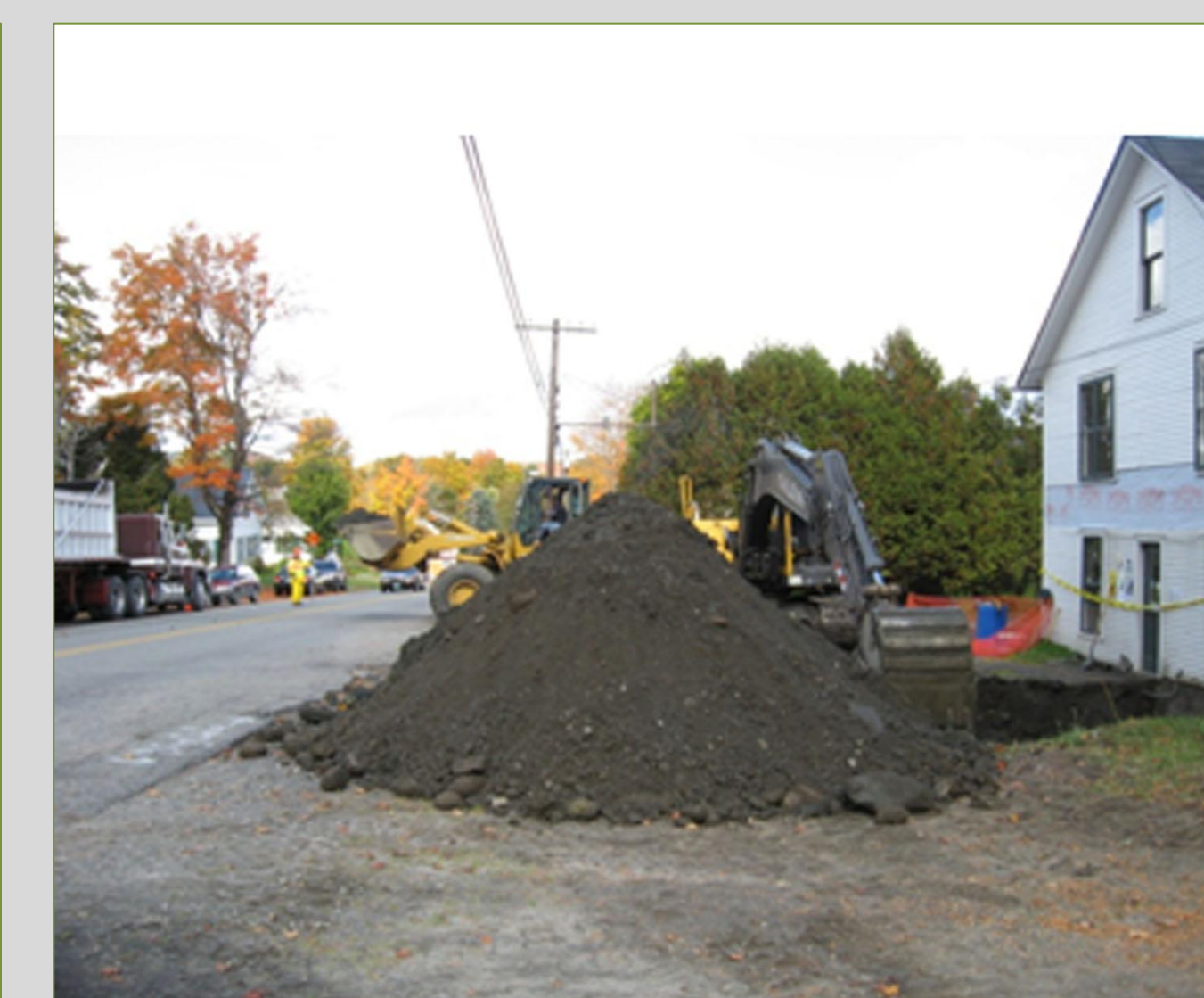
Soil Excavation and Loading
