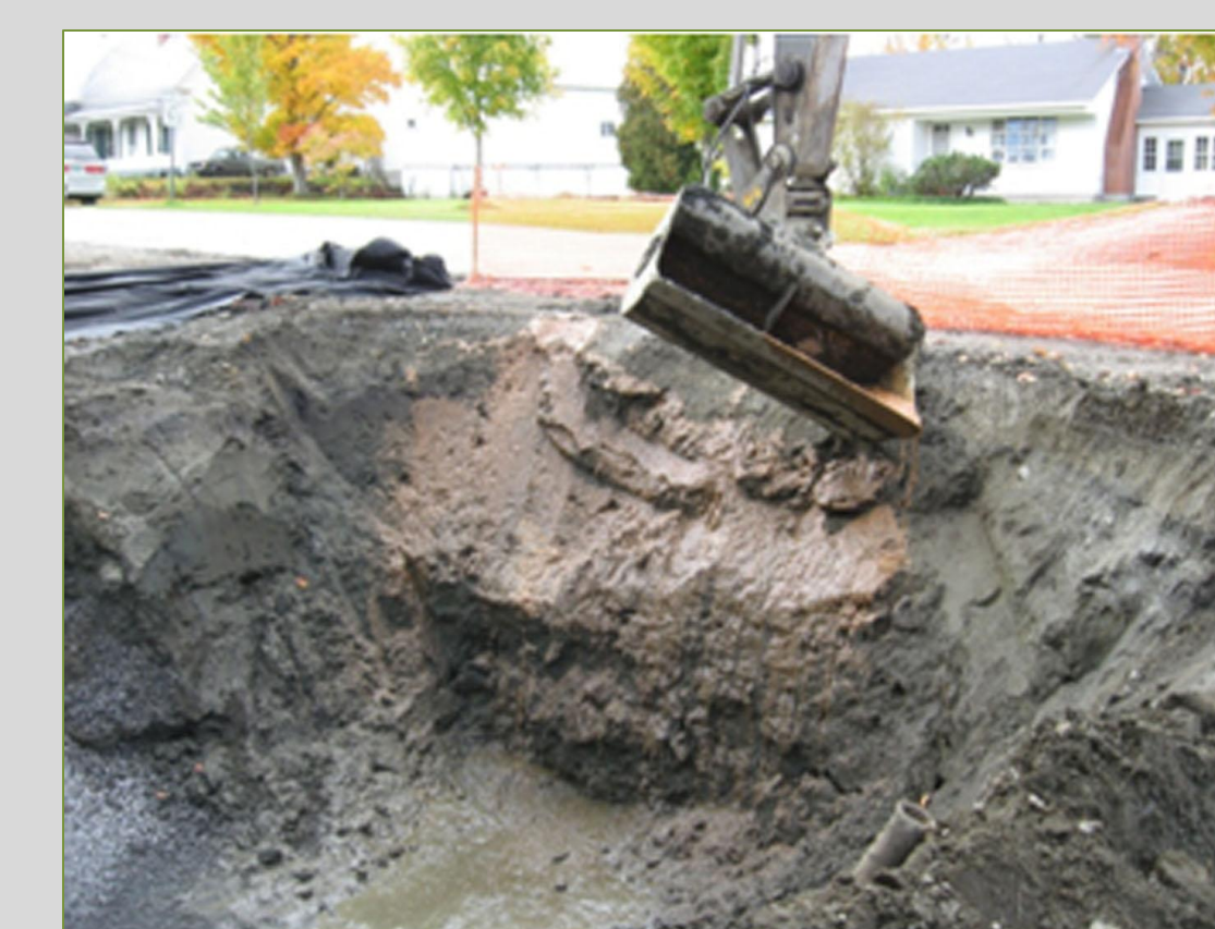
Application of RegenOx to Sidewalls and Base of Excavation
