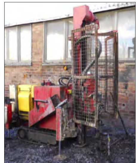
DP Injection Rig
