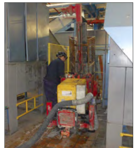
Indoor injection between dry cleaning machinery
