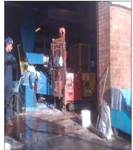
Injection Rigs weekend working within active laundry to minimise disruption
