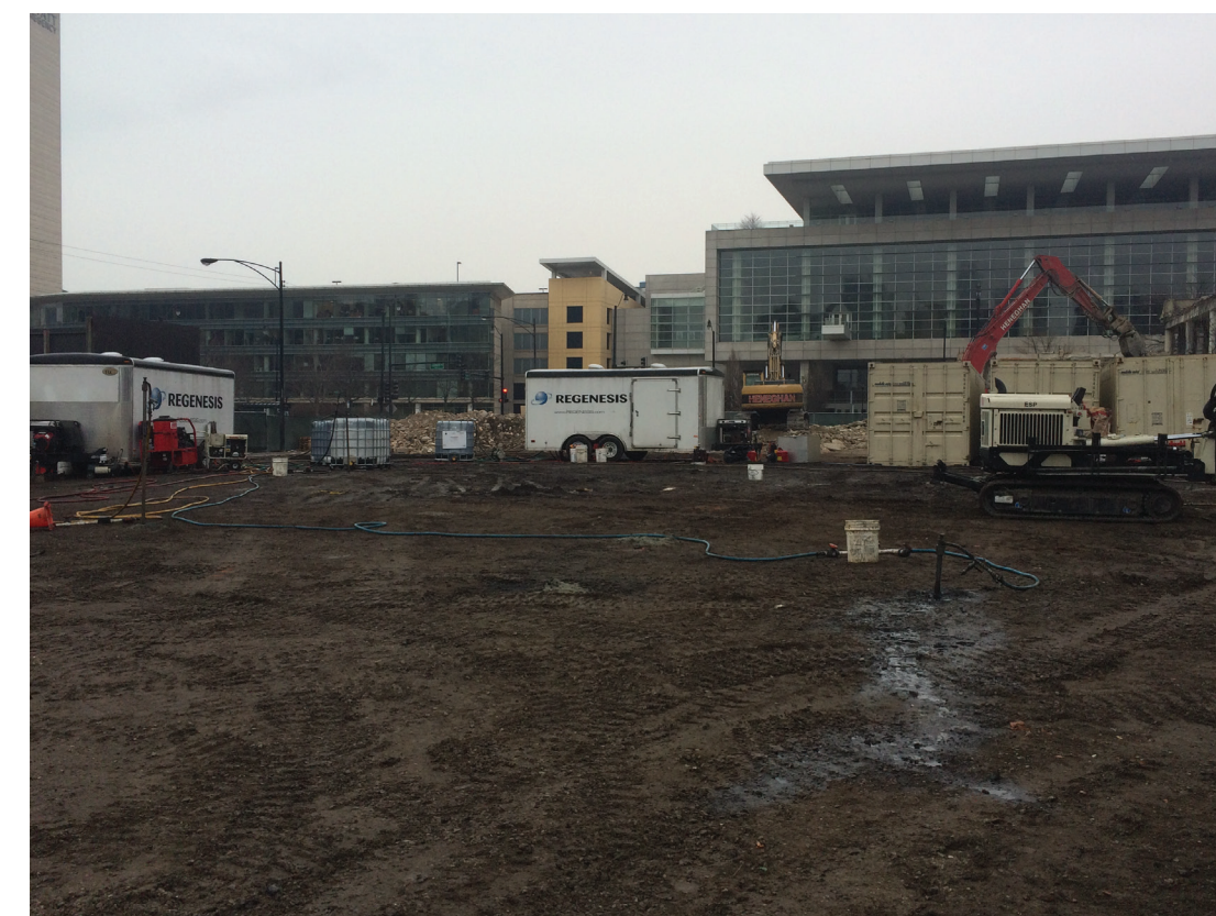
Project site during injection activities
