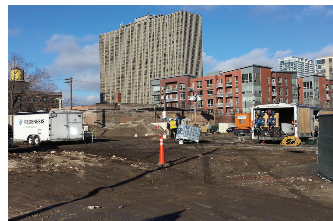
Project site during injection activities
