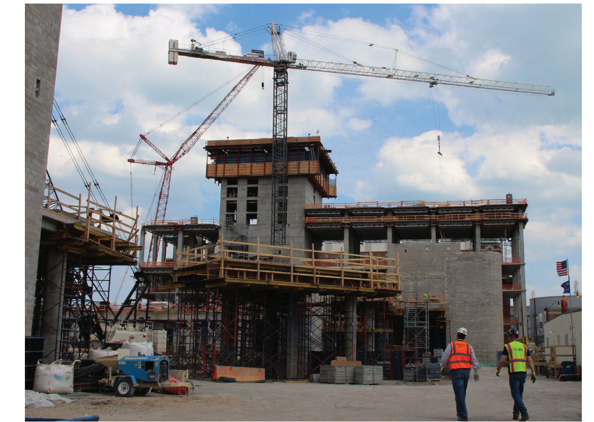
New construction on project site
