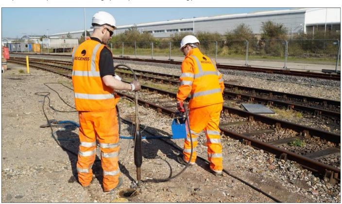
The first phase comprised the installation of a pump and treat (P&T) system enhanced with PetroCleanze in order to rapidly remove the LNAPL and adsorbed contamination in the smear zone. 18 treatment wells and 10 monitoring wells were installed across the target area: along the access road, the fuel point and within the four foot and six foot of the rail.
