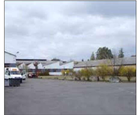
Fig. 3 The buildings and activity on the site made access difficult in some areas
