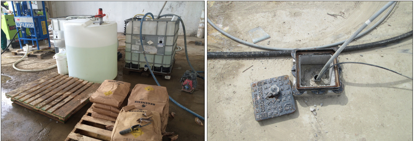
Fig. 5 and 6 Injection setup and multi-valve injection points
