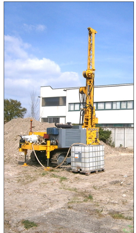
Fig. 1 Installation of injection points
