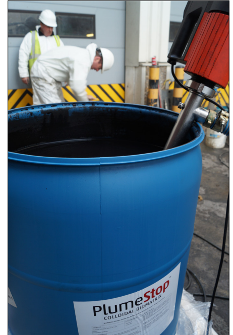
PlumeStop preparation for injection
