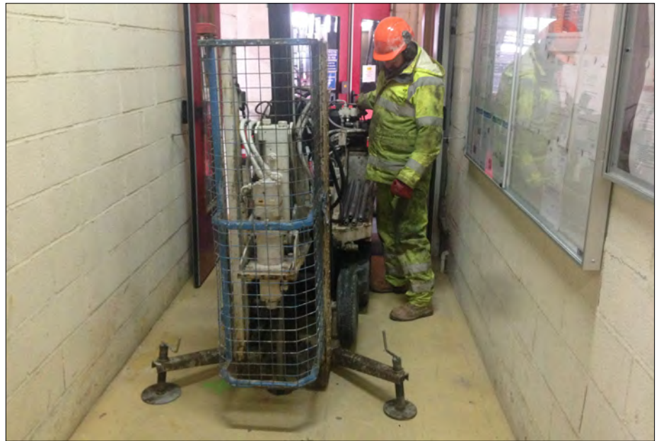
Fig. 4 Injection into downgradient plume in barrier formation, inside the factory building
