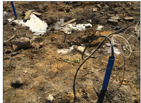
Fig. 3 Daylighting experienced in parts of the site
