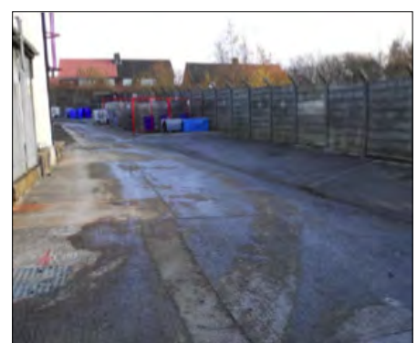
Remediation in full swing in the yard. Disturbance to business operations kept to a minimum
