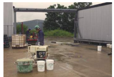
Fig. 5 - ORC-A pilot test application in Area A
