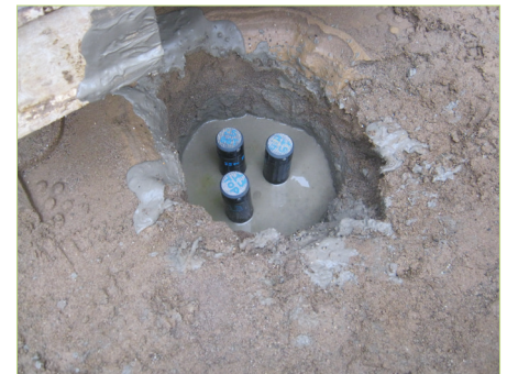
Fig.4: Nested injection wells as built
