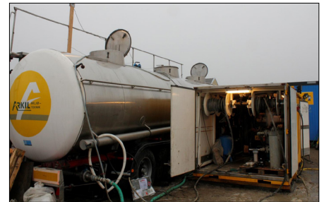
The heating of 3DMe to 40° prior to injection (photo: Arkil)
