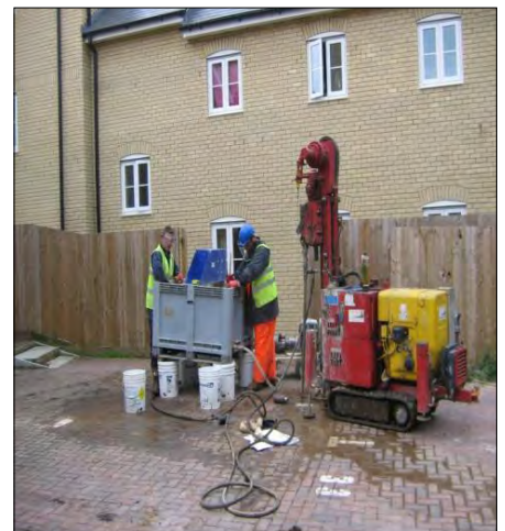
Figure 1: On site RegenOx injections using a direct push injection rig
