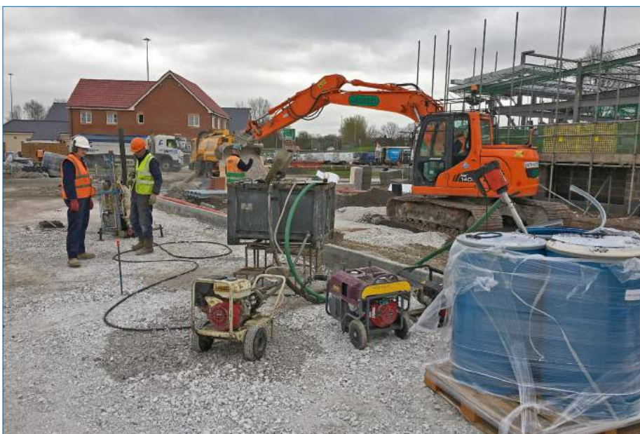
Fig. 12 - Injection of PlumeStop barrier by REGENESIS
