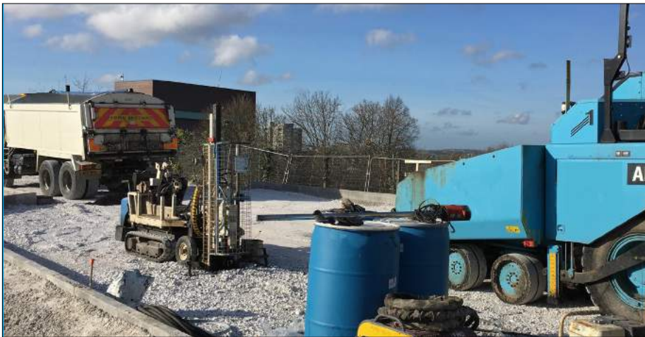
Fig. 1 - PlumeStop barrier injection near site boundary
