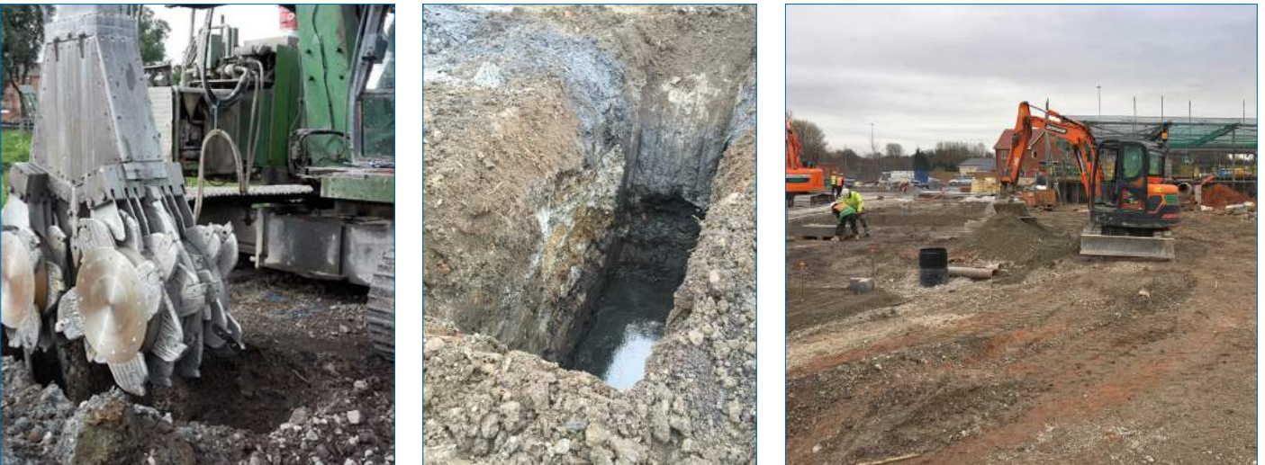
Fig. 9,10 and 11 - Installation of the soil-cement stabilisation panels by Deep Soil Mixing Ltd
