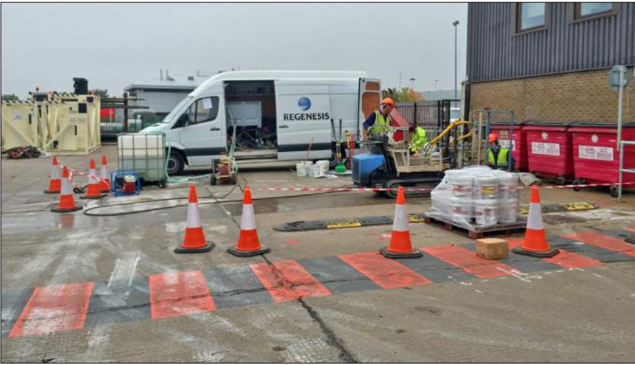
Fig. 1 REGENESIS Remediation Services applying 3DMe and BDI Plus on site
