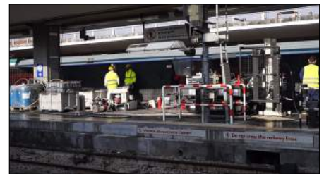
Fig. 5, Injection of PlumeStop on the platform of the railway station, in Area 3
