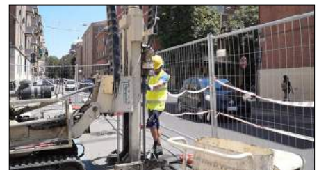
Fig. 6, Direct push injections in the road at Area 4
