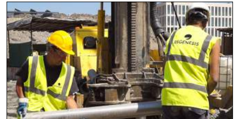
Fig. 4, Drilling wells prior to injection in Area 2
