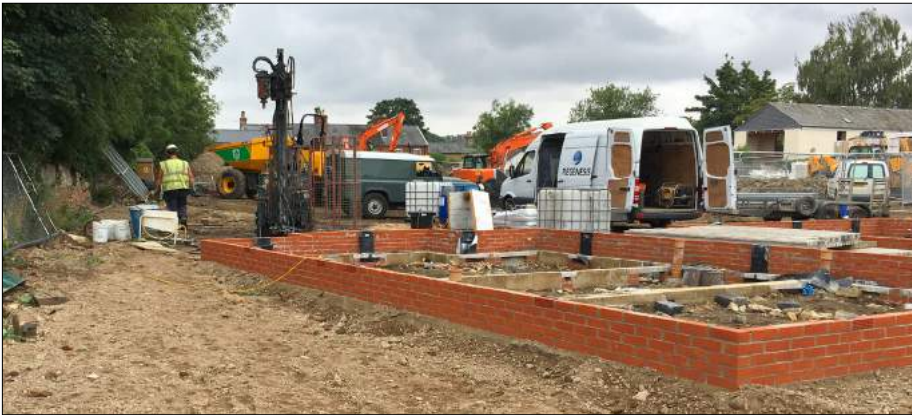
Fig. 1 - Remedial works at residential construction site
