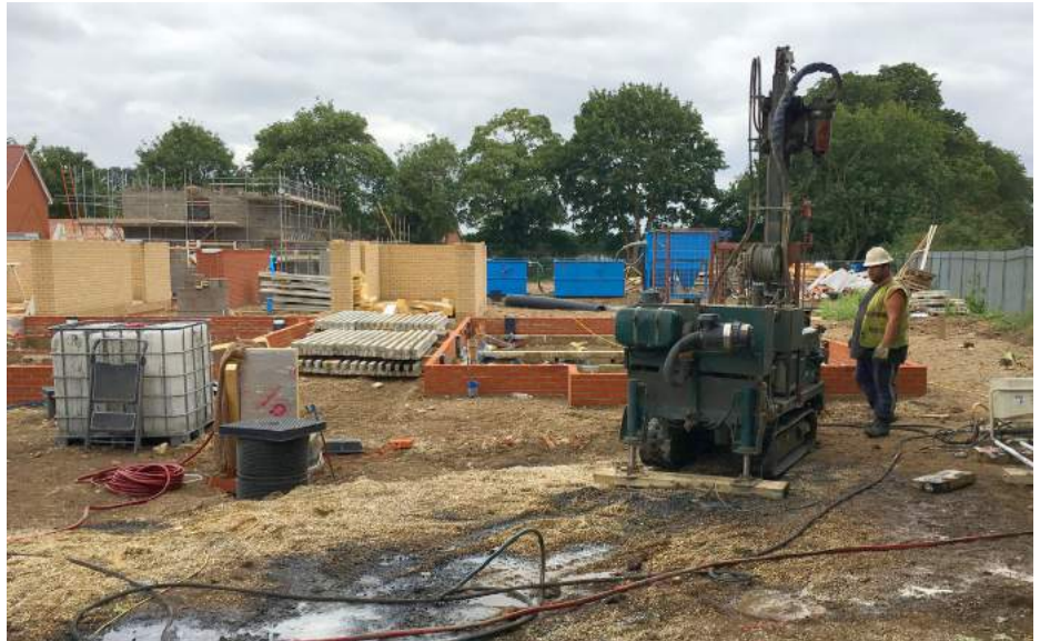
Fig. 4 - Bio piles, with in foreground the tubs of ORC Advanced Pellets, Fig. 5 - ORC Advanced slurry being prepared prior to injection, Fig. 6 - Geoprobe rig injecting reagents into the sub surface
