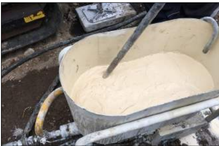
Fig. 4 - Bio piles, with in foreground the tubs of ORC Advanced Pellets, Fig. 5 - ORC Advanced slurry being prepared prior to injection, Fig. 6 - Geoprobe rig injecting reagents into the sub surface
