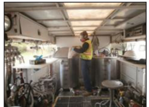
3,000 pounds of ORC Advanced was mixed and applied on-site.
