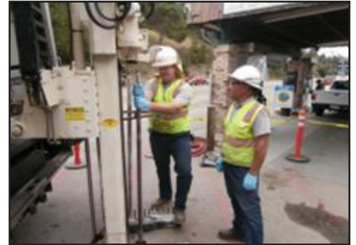
14 direct-push injection points were used to apply the product.
