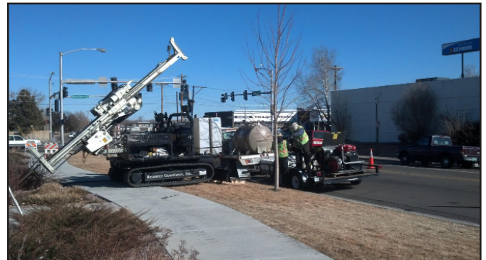
Angled injections were required to apply ORC Advanced beneath the active restaurant.
