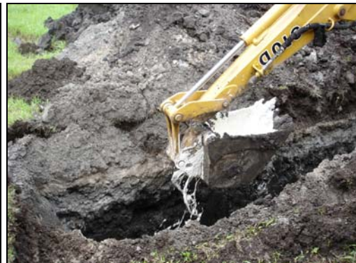
Figure 3. ORC Advanced® Slurry Applied to Trenches
