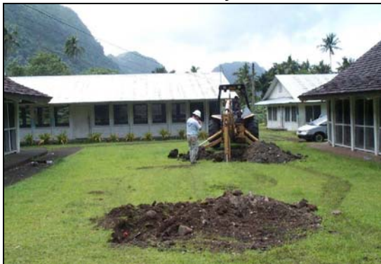
Figure 2. Trench Construction at the Elementary School
