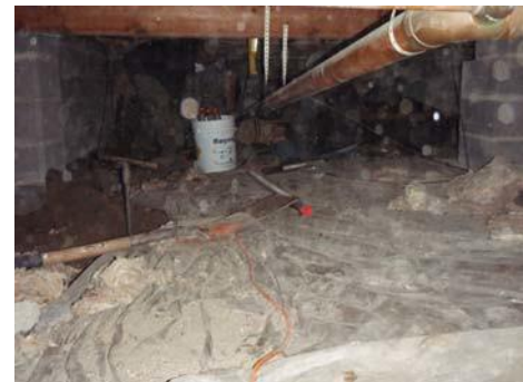
Figure 2. Crawl Space Injection Point
