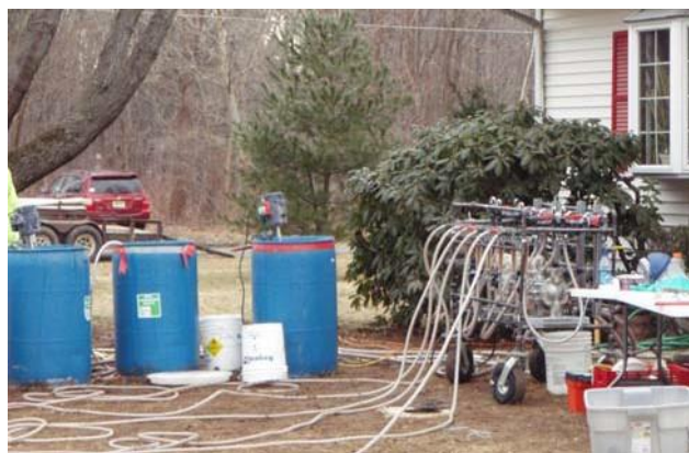
Figure 3. Specially Designed Injection System Applied Six Points Simultaneously
