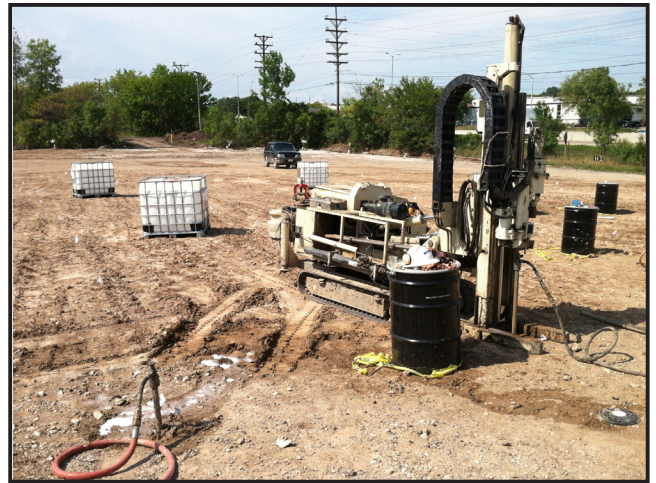
10-foot vertical injections were applied into silty sand and clay over weathered bedrock.
