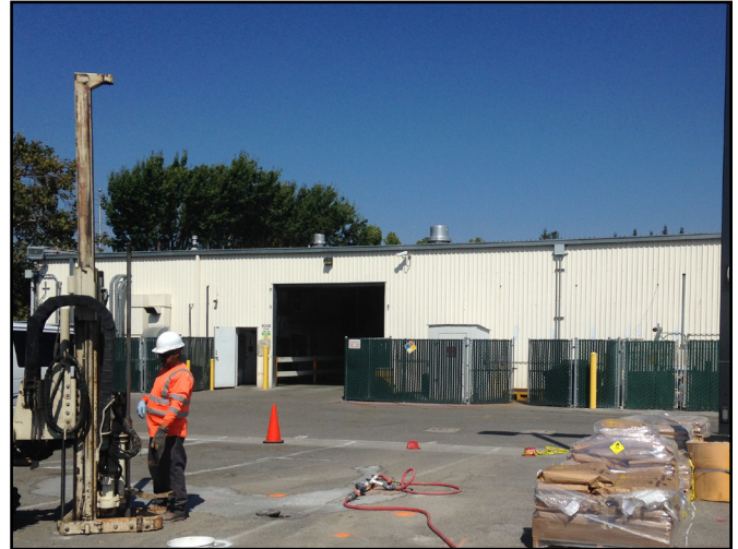
RegenesiS Remediation Services applied PersulfOx into low permeability soils without surfacing.
