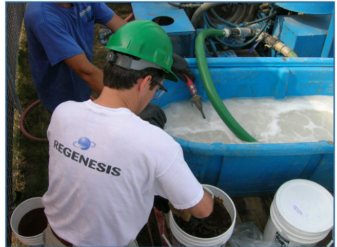
PersulfOx was applied sub-slab near the source to inhibit vapor issues within the building.
