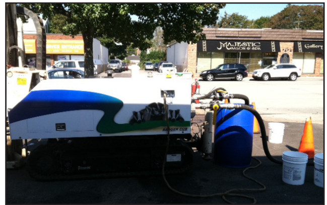
A Badger Injection System, operated by Environmental Assessment and Remediation, was used on-site.
