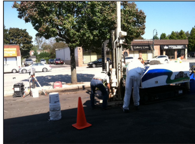
RegenOx was applied to three Long Island sites that were heavily impacted with BTEX.
