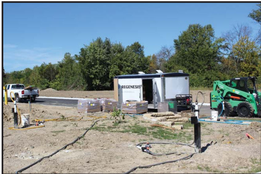
RegenesiS Remediation Services applied PersulfOx at four areas on-site.
