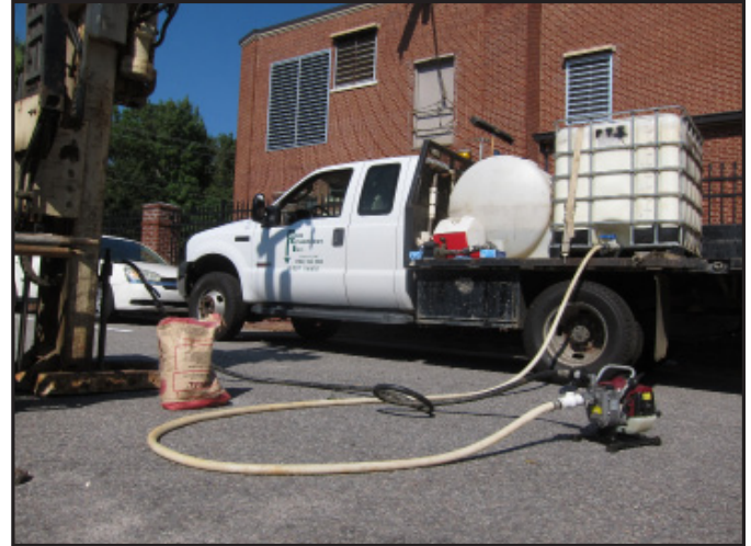
3-D Microemulsion was applied on-site to treat high PCE concentrations.
