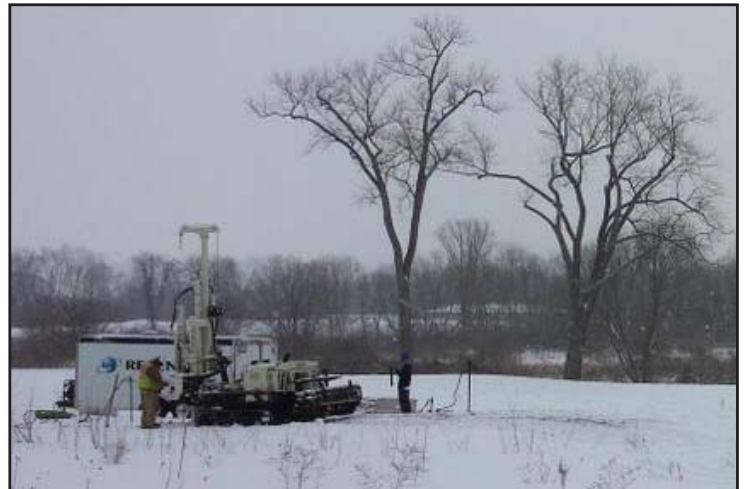
RRS applies combined remedies in freezing temperatures.
