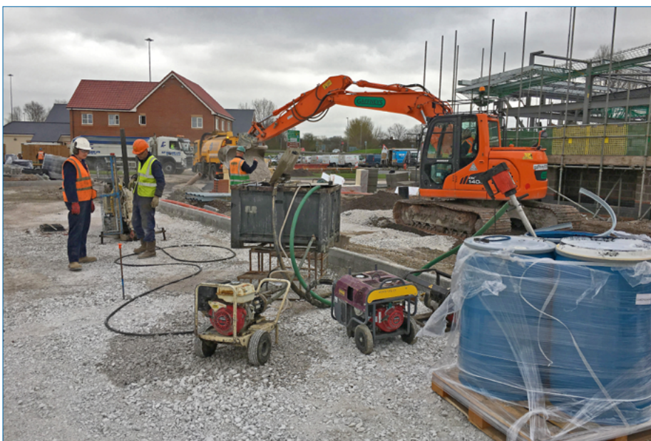
Fig. 12 - Injection of PlumeStop barrier by REGENESIS
