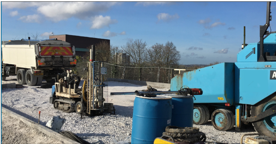
Fig. 1 - PlumeStop barrier injection near site boundary
