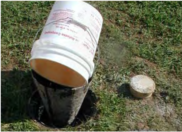
Fig. 4 HRC being gravity-fed into one of the application wells
