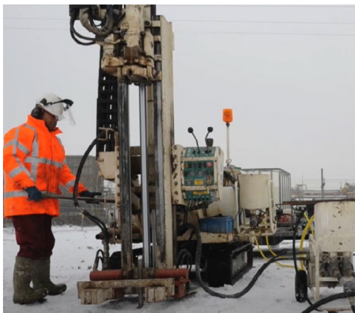
Fig. 1 Direct push injection of 3DME
