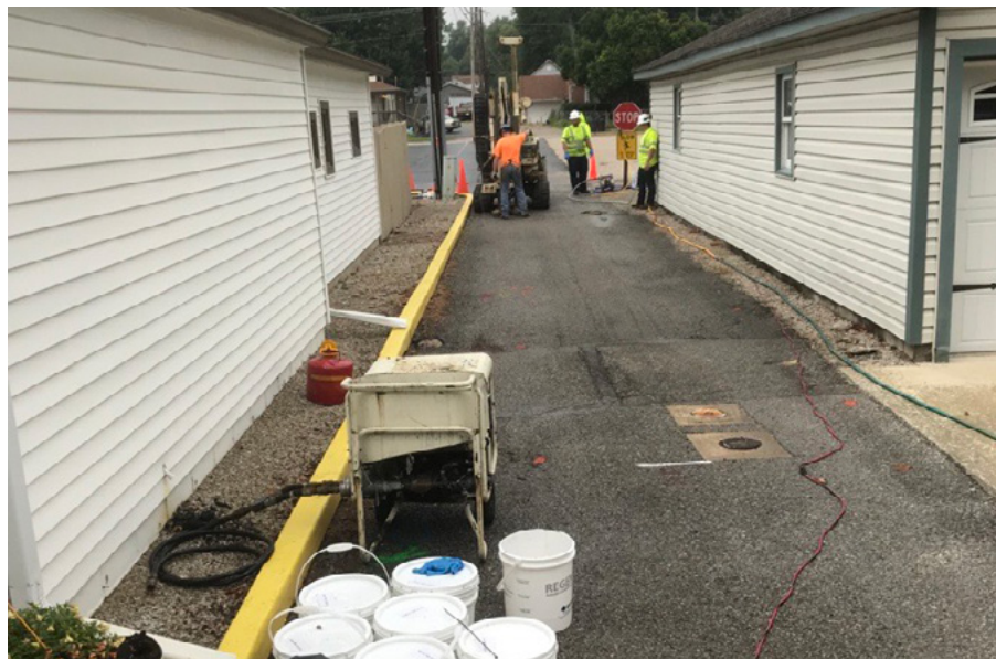
Workers applying amendments at IP-10 in July 2017
