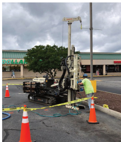
Uni-Tech Drilling injects PetroFix Remediation Fluid into the soil using a GeoProbe
