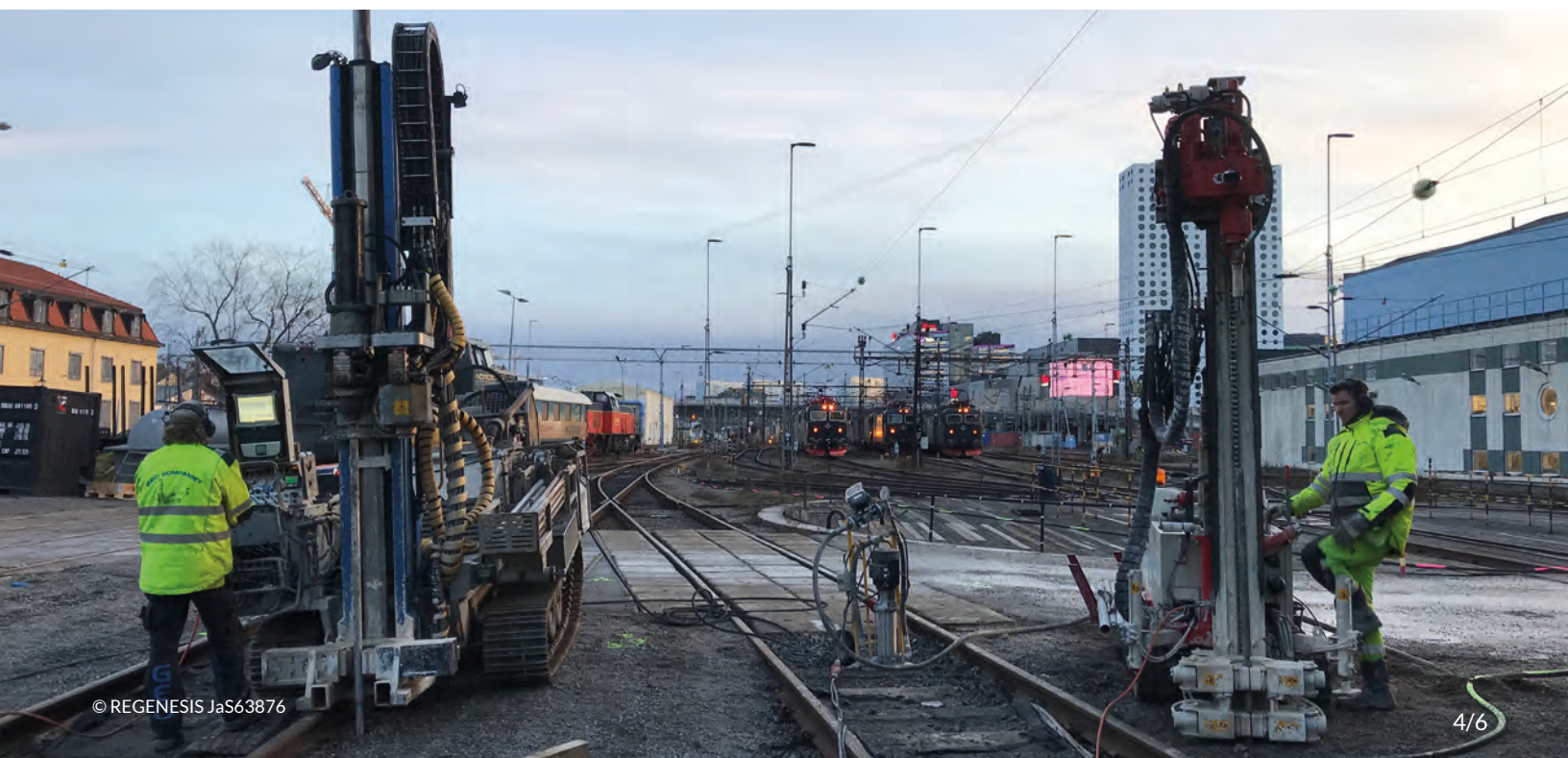
Top: PetroFix, RegenOx and ORC-Advanced storage onsite. Above: Envytech's reagent mixing setup. Below: Direct Push Injection rigs in action.
