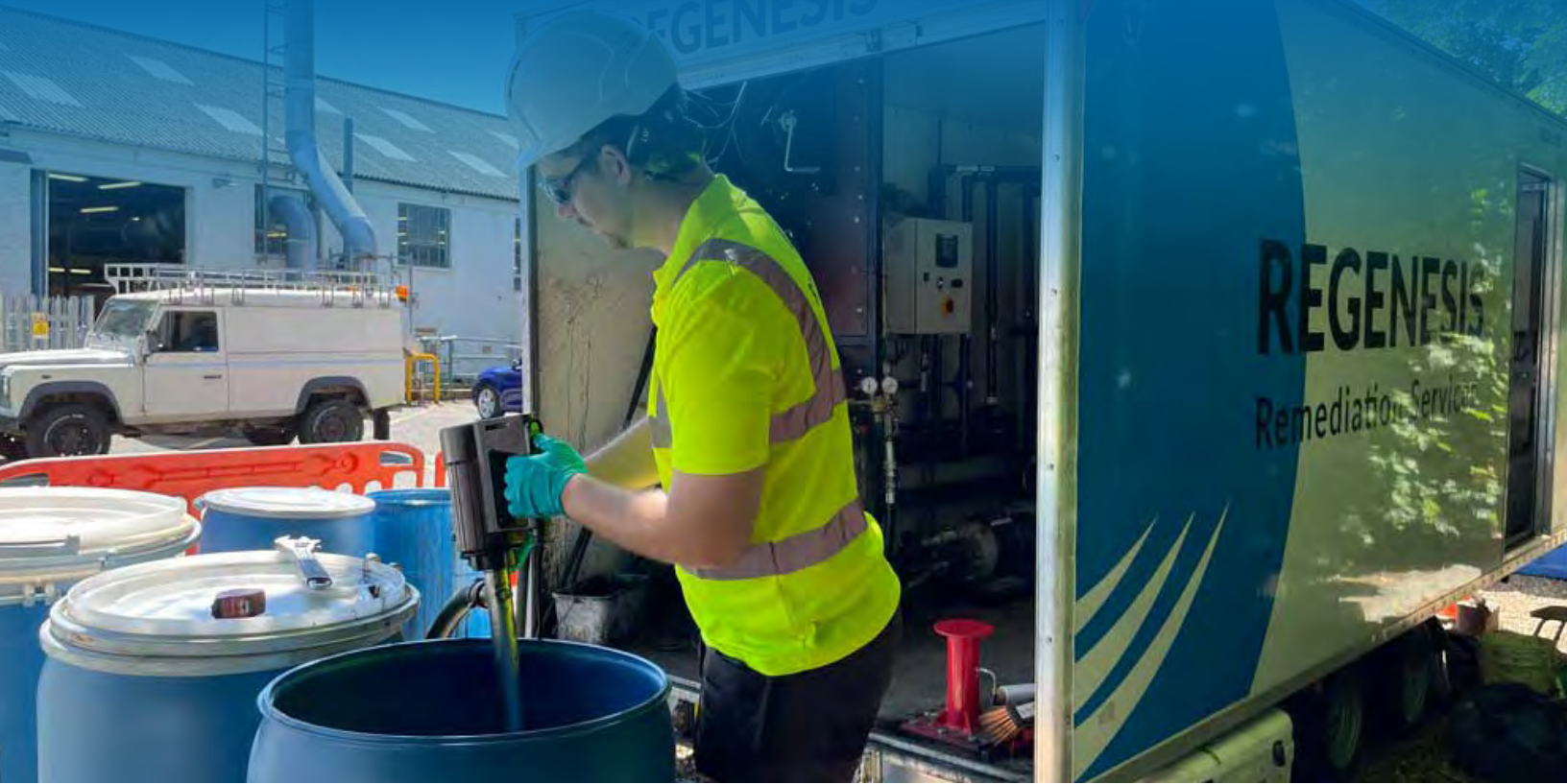
Fig. 10 REGENESIS' mobile mixing station was used in the full-scale remediation works
