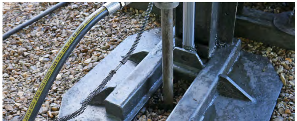
Fig. 6-9 Details of the pilot trial undertaken by REGENESIS Remediation Services
