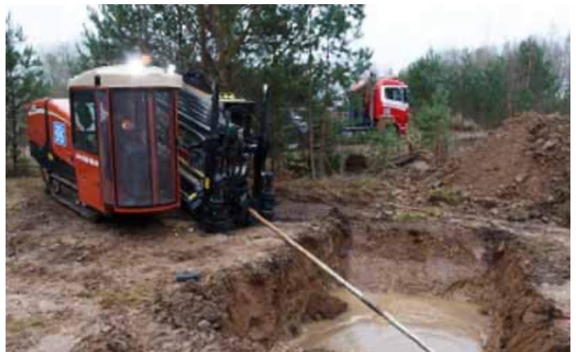
Fig. 3 and 4 Remediation works on site, including directional injection ©RGS Nordic
